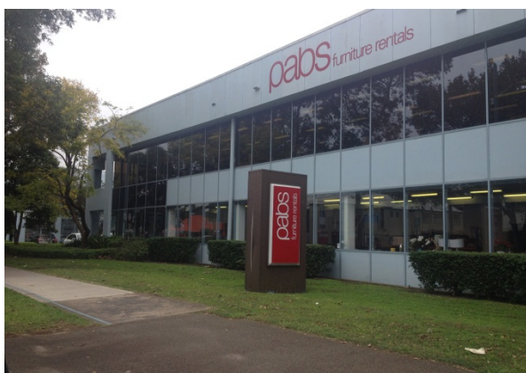
Figure 5.105: An example of a landscaped setback that presents well to the street and softens the appearance of the building
